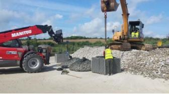
3 Plifting ring. Lift slightly to bind the top of the bag.
