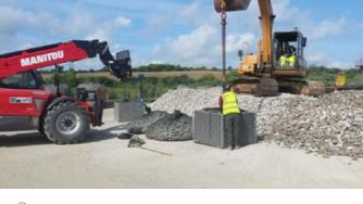
⑤Lift up the filling frame and leave the Filter Unit.
